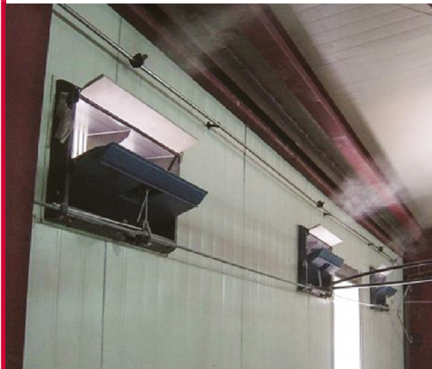
Figure 112 Example fogging system for a cross-ventilated house.
