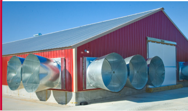
Figure 107 Example of a typical tunnel-ventilated house.
