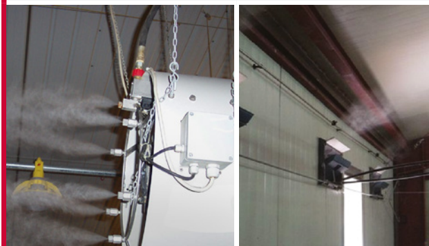
Figure 15 Use of a mister to increase RH during brooding.
