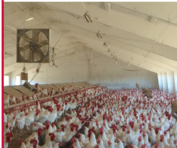
Figure 96 Circulation fans in an open-sided/naturally ventilated house.
